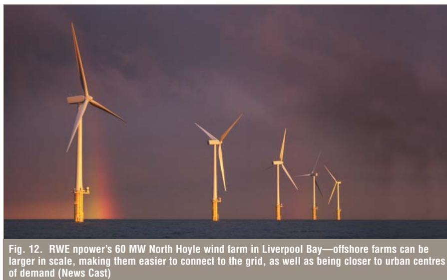
Fig. 12. RWE npower's 60 MW North Hoyle wind farm in Liverpool Bay—offshore farms can be larger in scale, making them easier to connect to the grid, as well as being closer to urban centres of demand (News Cast)
