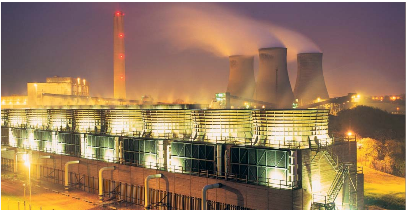
Fig. 5. RWE npower's Didcot B combined-cycle gas turbine power station with Didcot A coal-fired station behind—these two types of power station currently provide around 75% of UK electricity and need to be maintained and renewed (News Cast)
